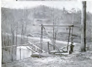
One of the wells, with the rocking-lever mechanism that transforms the cable pull into straight-line motion for the pump. The engine house is seen on the distant hill
